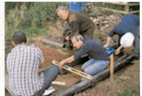
Building the extension
